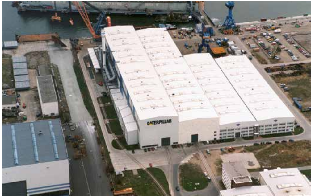
Picture: Caterpillar Motoren Rostock GmbH.
