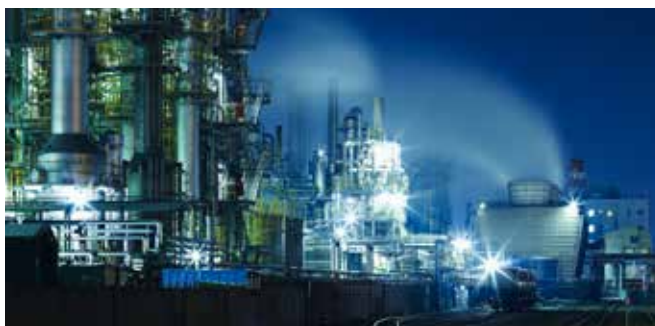
Oil and gas. Consumption measurement for gas turbines.
