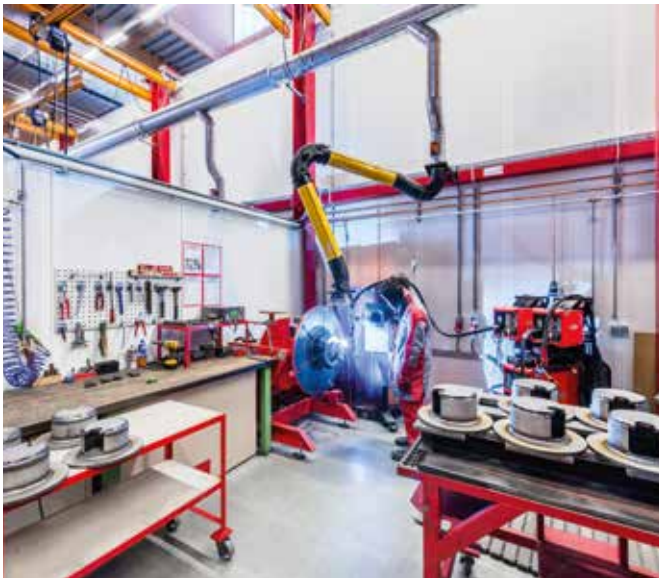
One of five modern welding booths.
